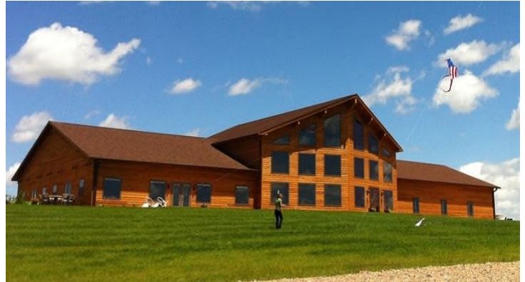
Photo of Calico Skies Winery & Vineyard in southwest Lyon County
