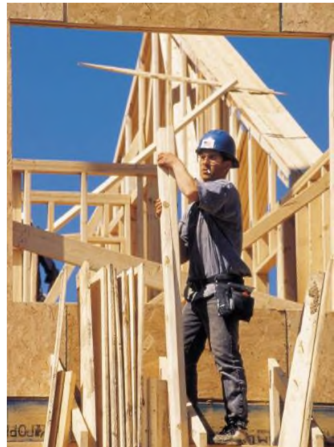
Photo of a house under construction
